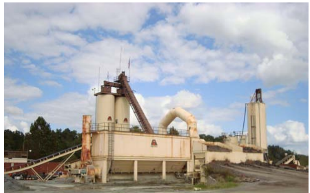
The asphalt plant.
