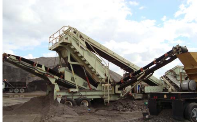
Screener and four (4) conveyor belts.
