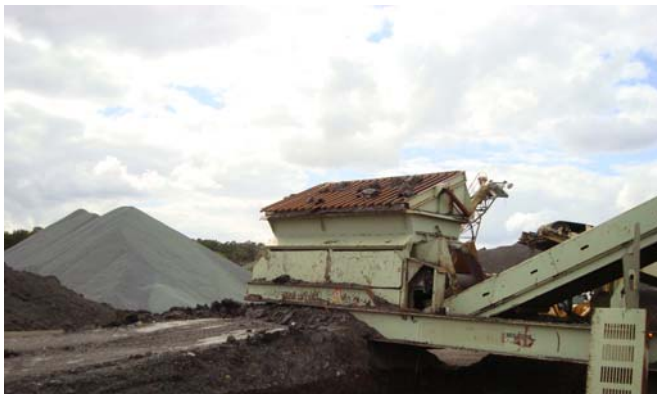
Loader for the crusher with initial screener.
